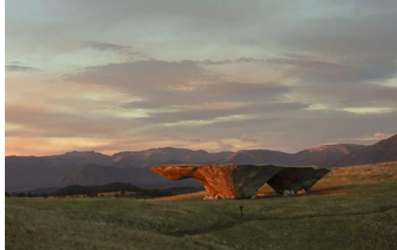
The Domo is one of the outdoor music venue's that creates a raw environment for visitors of Tippet Rise to experience music. (Photo by Kevin Kinzley. Courtesy of Tippet Rise Art Center.)
