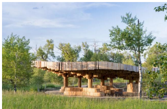
Pritzker Prize-winning architect Francis Kéré designed Xylem, a permanent pavilion built from the wood of local ponderosa and lodgepole pines. Credit...Iwan Baan/Tippet Rise Art Center
