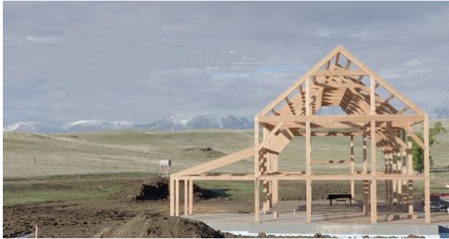
The Olivier Barn at Tippet Rise Art Center, under construction
